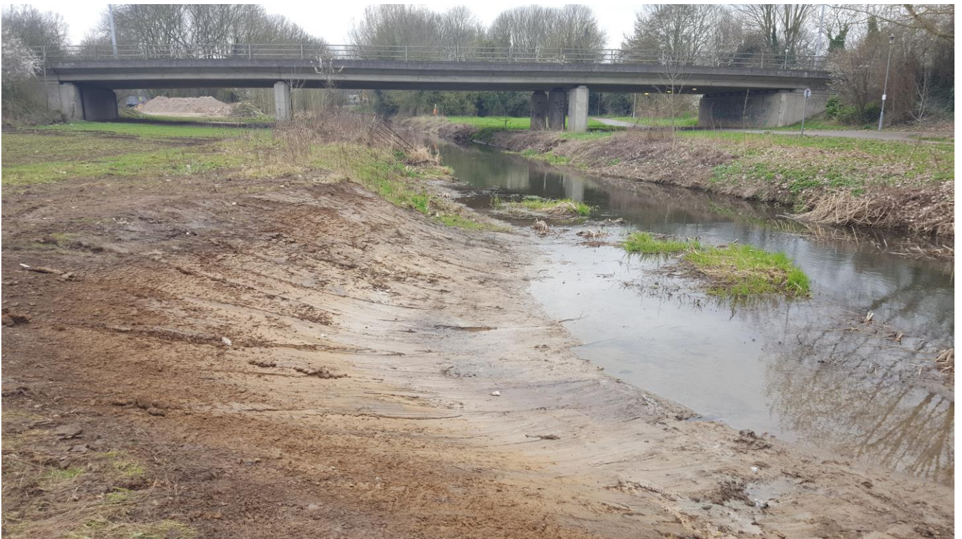
Photograph 3: The new fish refuge bay created at Springfield Nature Reserve, for fry and small fish to shelter away from the main river flow.
