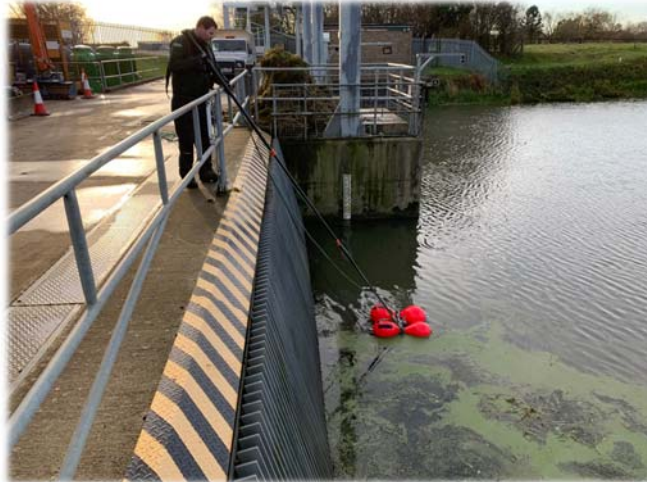
Figure 3 Officer Finnie operating scanning equipment at Peakirk Pumping Station
