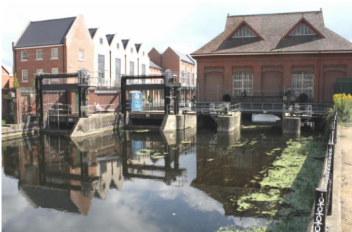
New Mills Pumping Station (Upstream)
